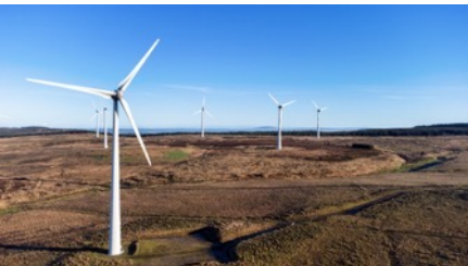
Average onshore wind turbine requires 300 tonnes of steel
