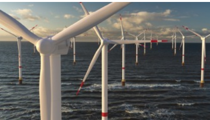
Average offshore wind turbine requires 1,800 tonnes of steel
