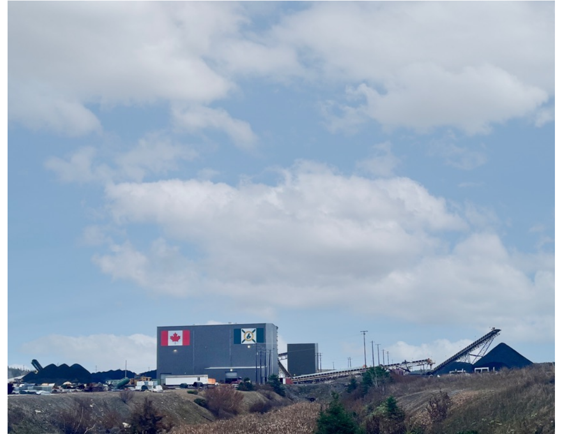
Donkin Mine, Oct 6, 2022. Coal washplant in foreground. Run-of-mine coal being stockpiled to the left of the washplant and a growing stockpile of washed coal to the right.
