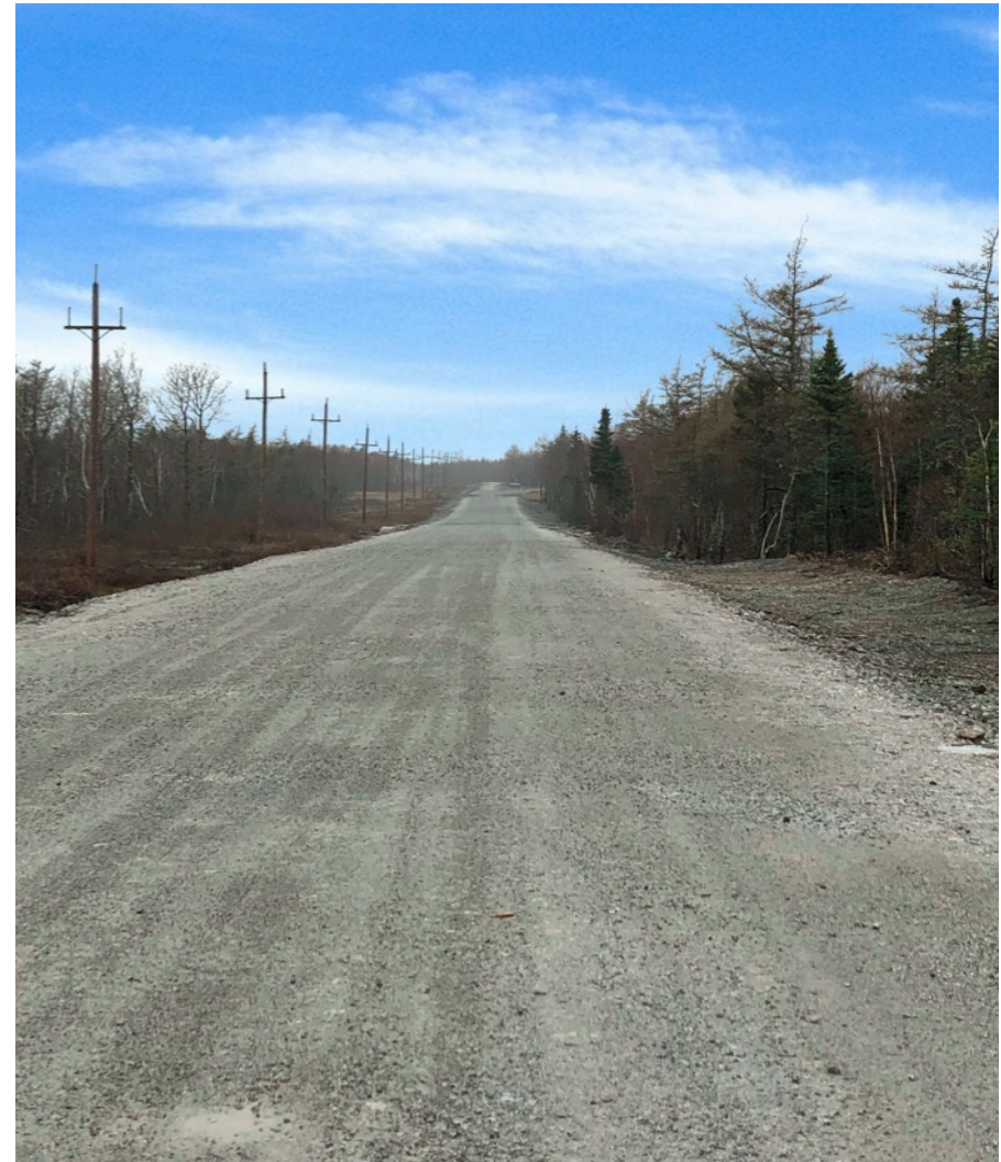
Kameron's private haul road is expected to be complete in 2019
