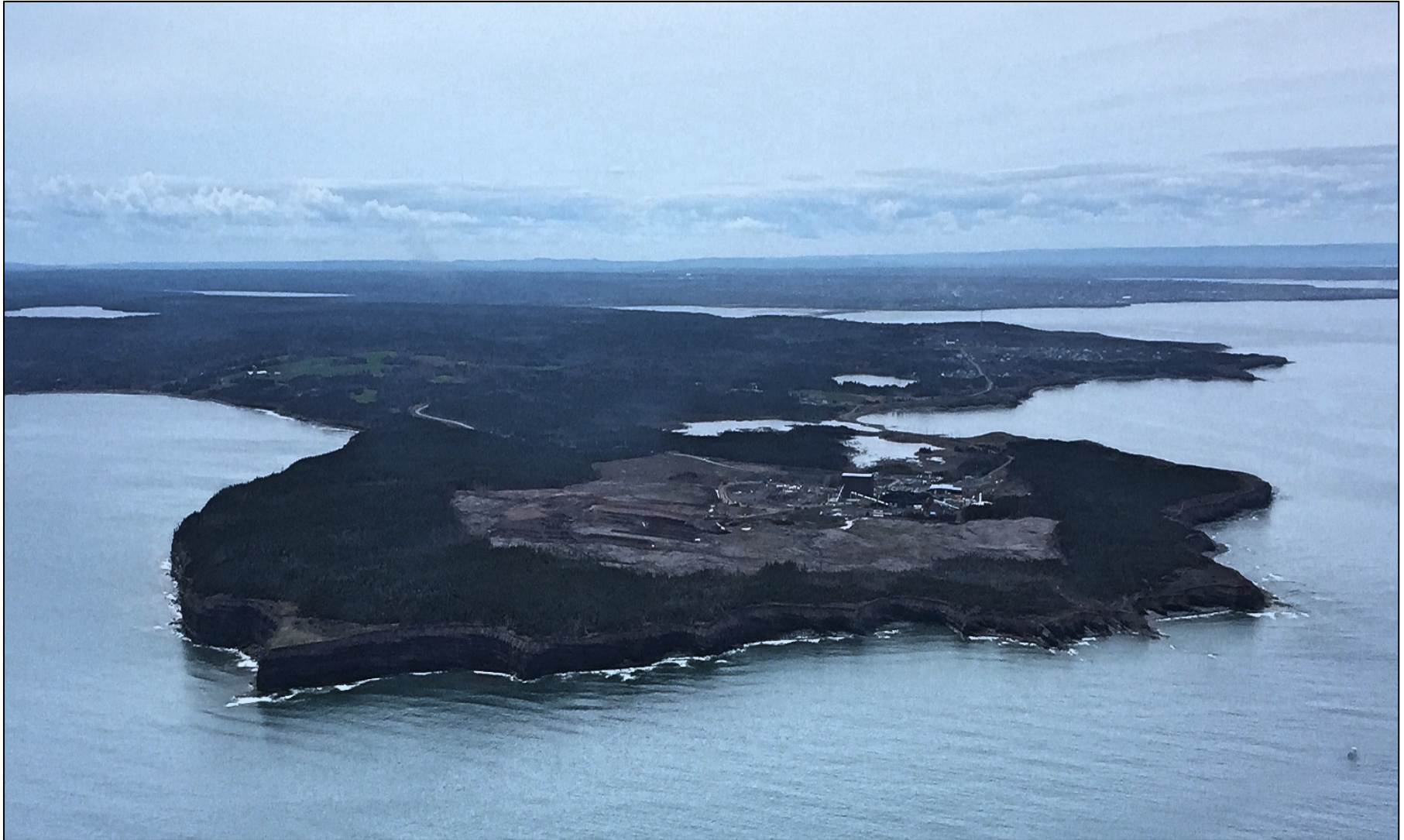
Donkin Coal Project. Photo taken May 2017
