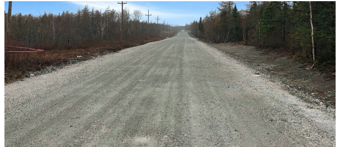
Kameron's private haul road
