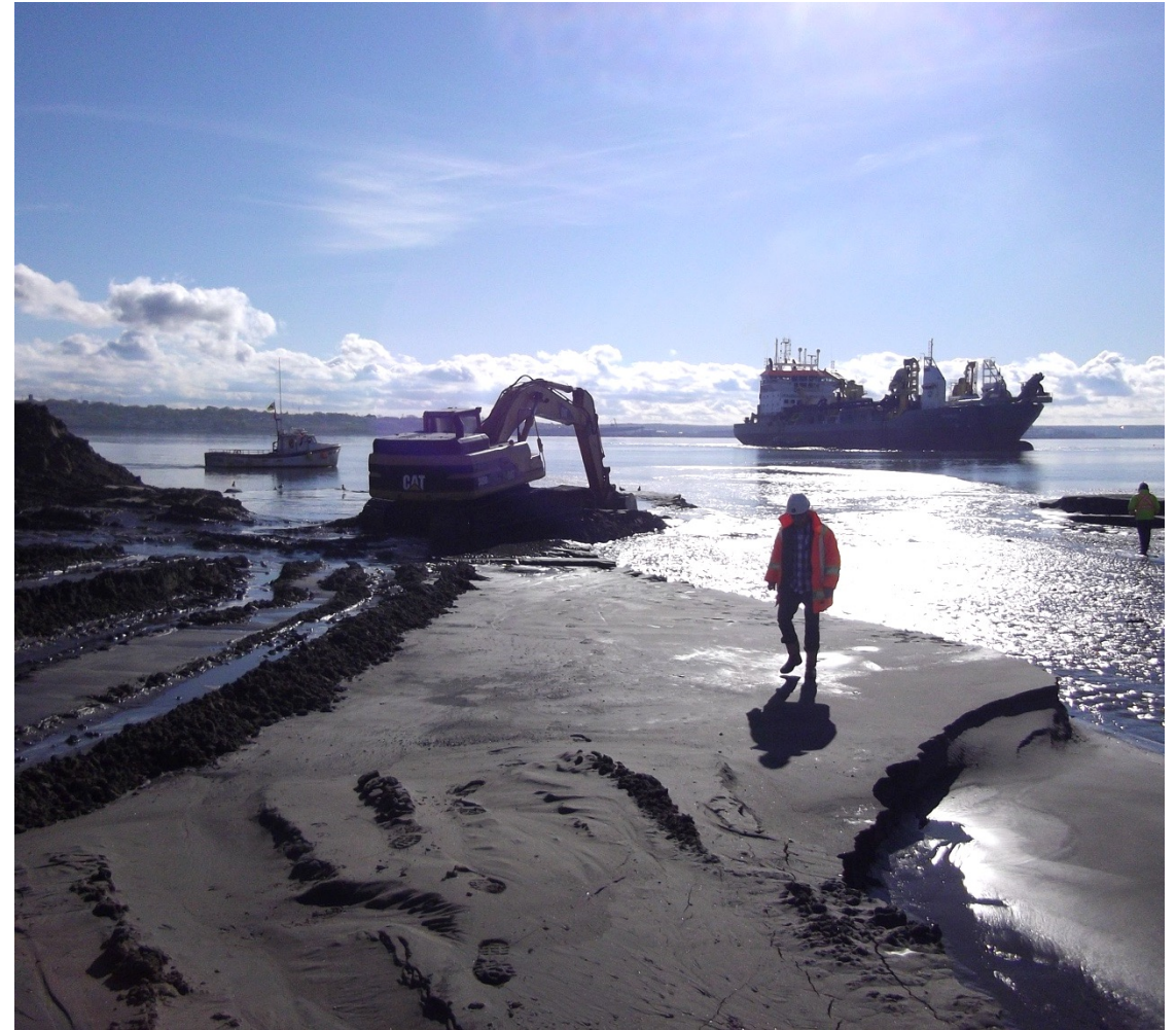
Dredge vessel at work in Sydney Harbour in 2011 (archived photo courtesy of CBCL Limited)
