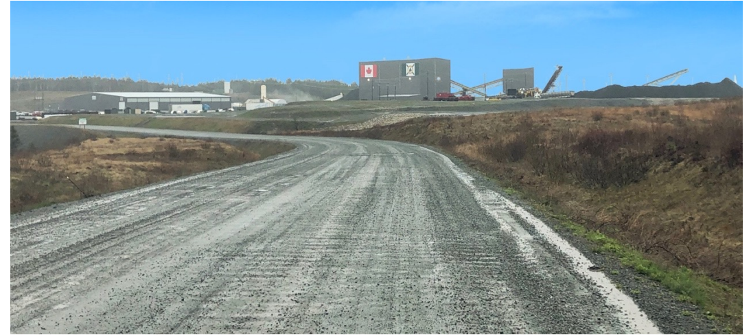
Donkin Mine surface infrastructure.
