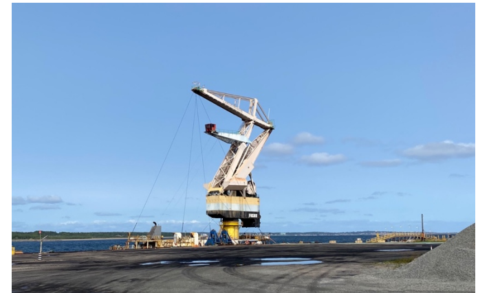
Recently delivered shiploader at PEV coal terminal
