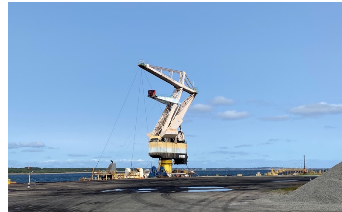
Recently delivered shiploader at PEV coal terminal
